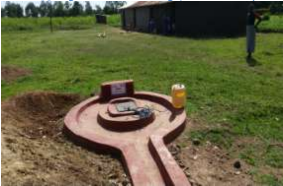
Well D293 dug for Nakhaliro village, Western Kenya.
