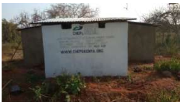
Completed latrines handed over to the school
