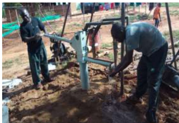
Completed borehole at Chakama Primary School
