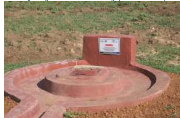
Well D290 dug for Kabukoshe village, Western Kenya.
