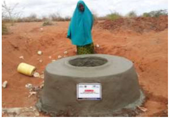
Well D281 dug for Markaba Muhumed of Bangal village
