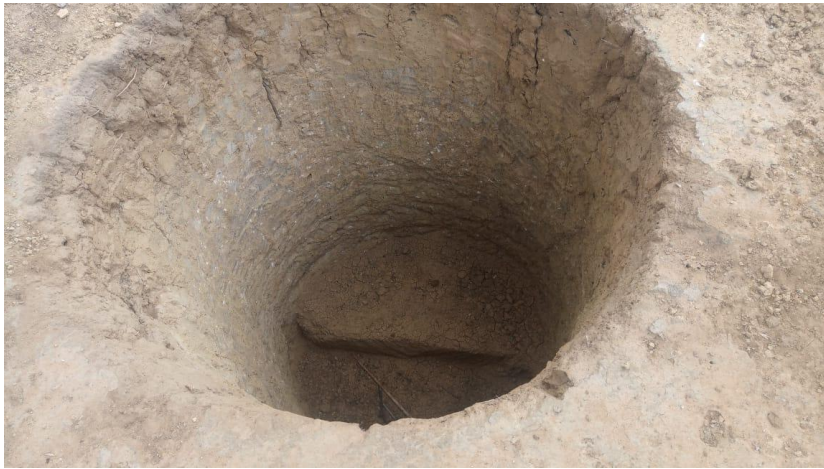
Pit hole for the latrines
