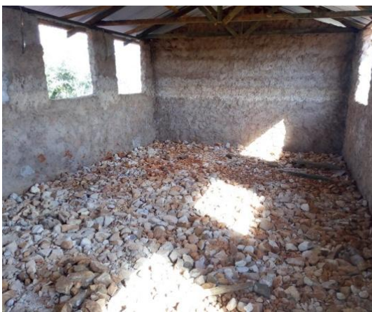
Images of the incomplete classrooms with un-plastered walls and floor
