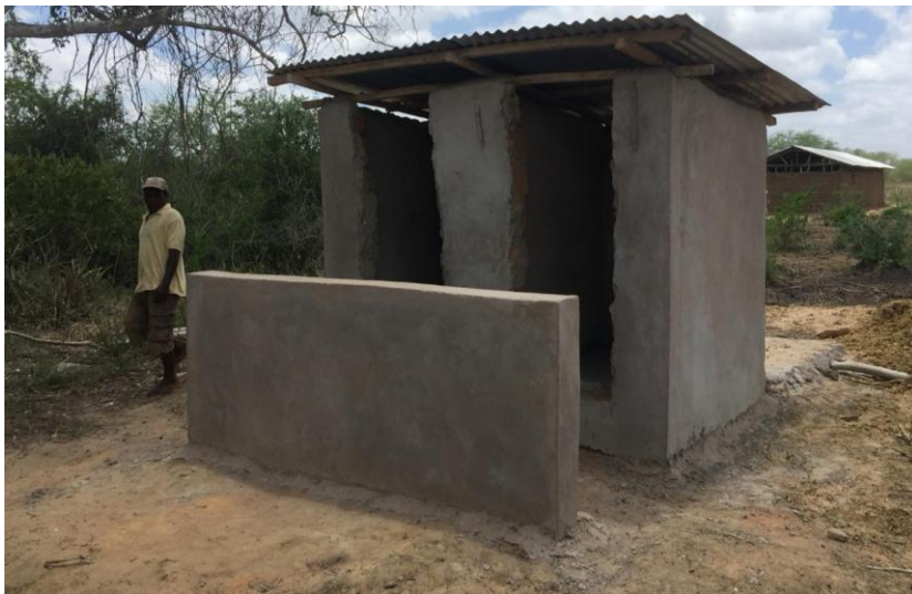
Construction in progress
