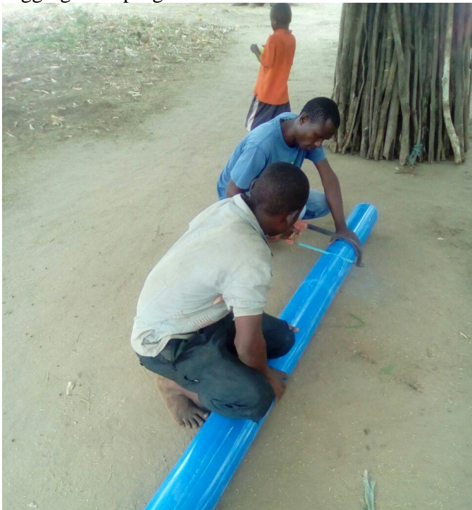
Cutting of pipe prior to fitting
