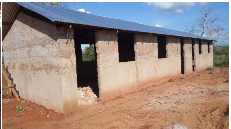
Images of the incomplete classrooms with un-plastered walls and floor
