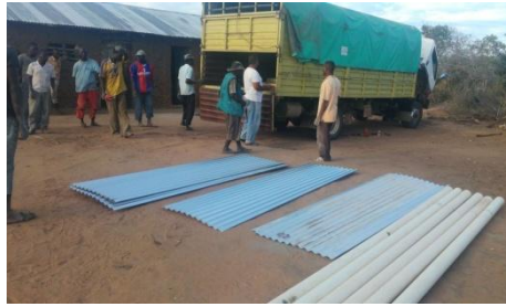
Delivery of construction material
