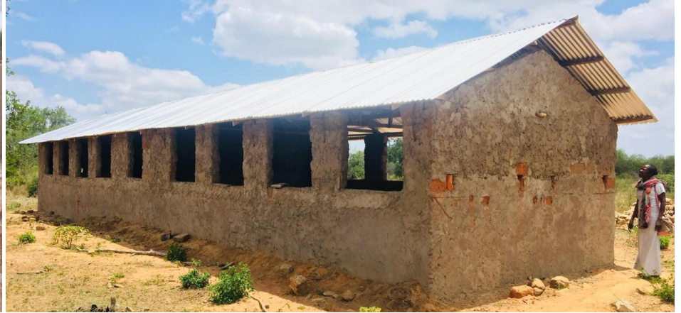
Construction in progress
