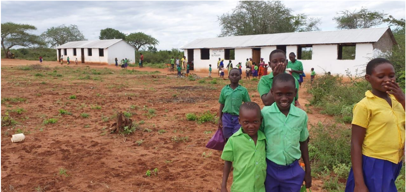
The two complete blocks of classrooms adjacent to each other
