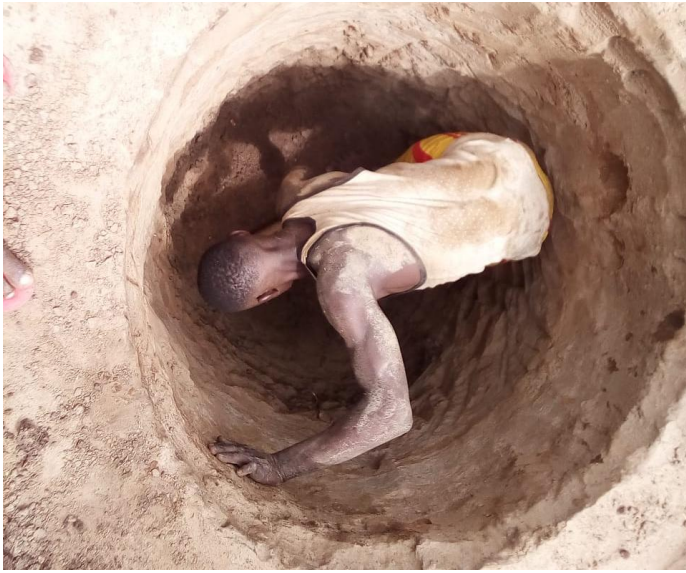
Digging in progress
