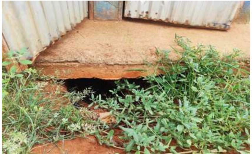
The only latrine in the entire school used by female students. Photo on the right shows its collapsing floor
