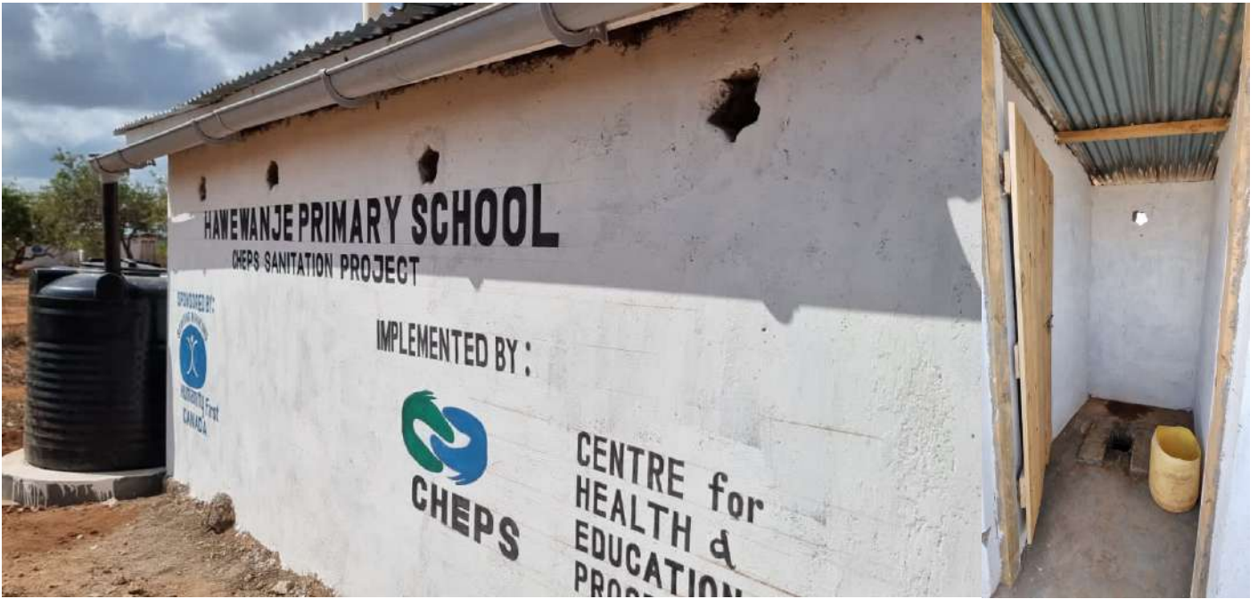
Two blocks of latrines constructed for boys and girls each, complete with rain harvesting and hand washing facilities
