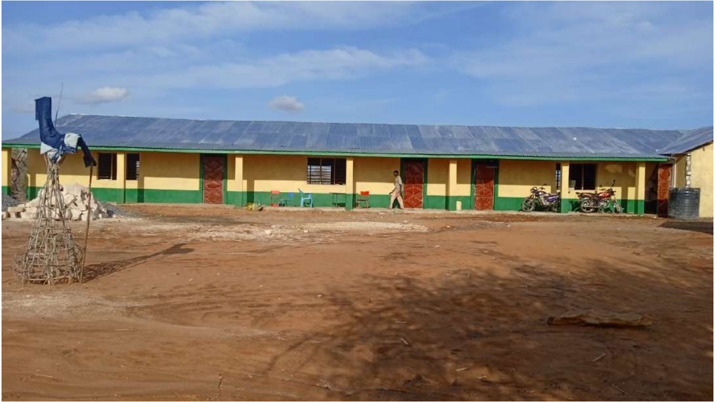
4 new classrooms completed
