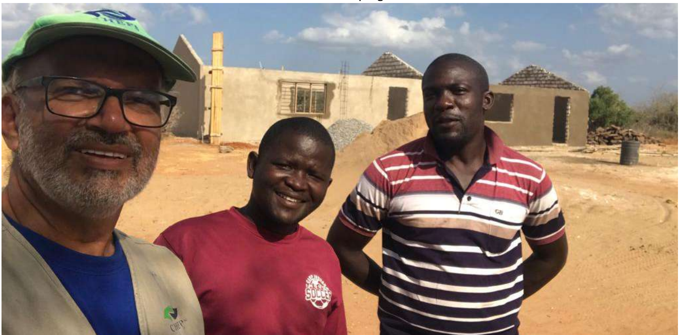
CHEPs CEO Dr. Muhsin Sheriff visiting the site to inspect progress.
