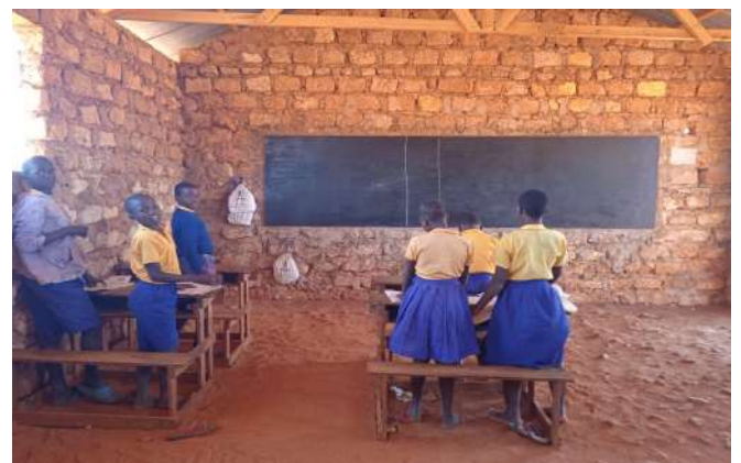
Students delighted to have a roof and blackboard in their classroom
