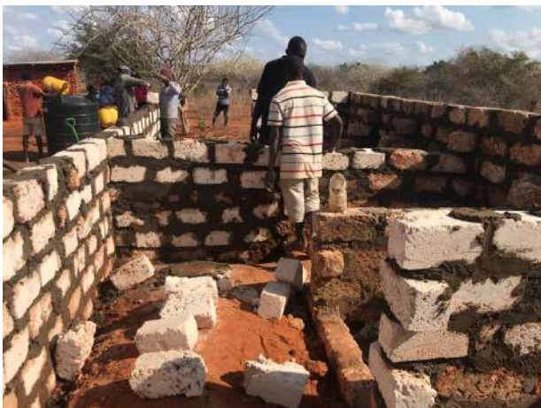
Construction in progress
