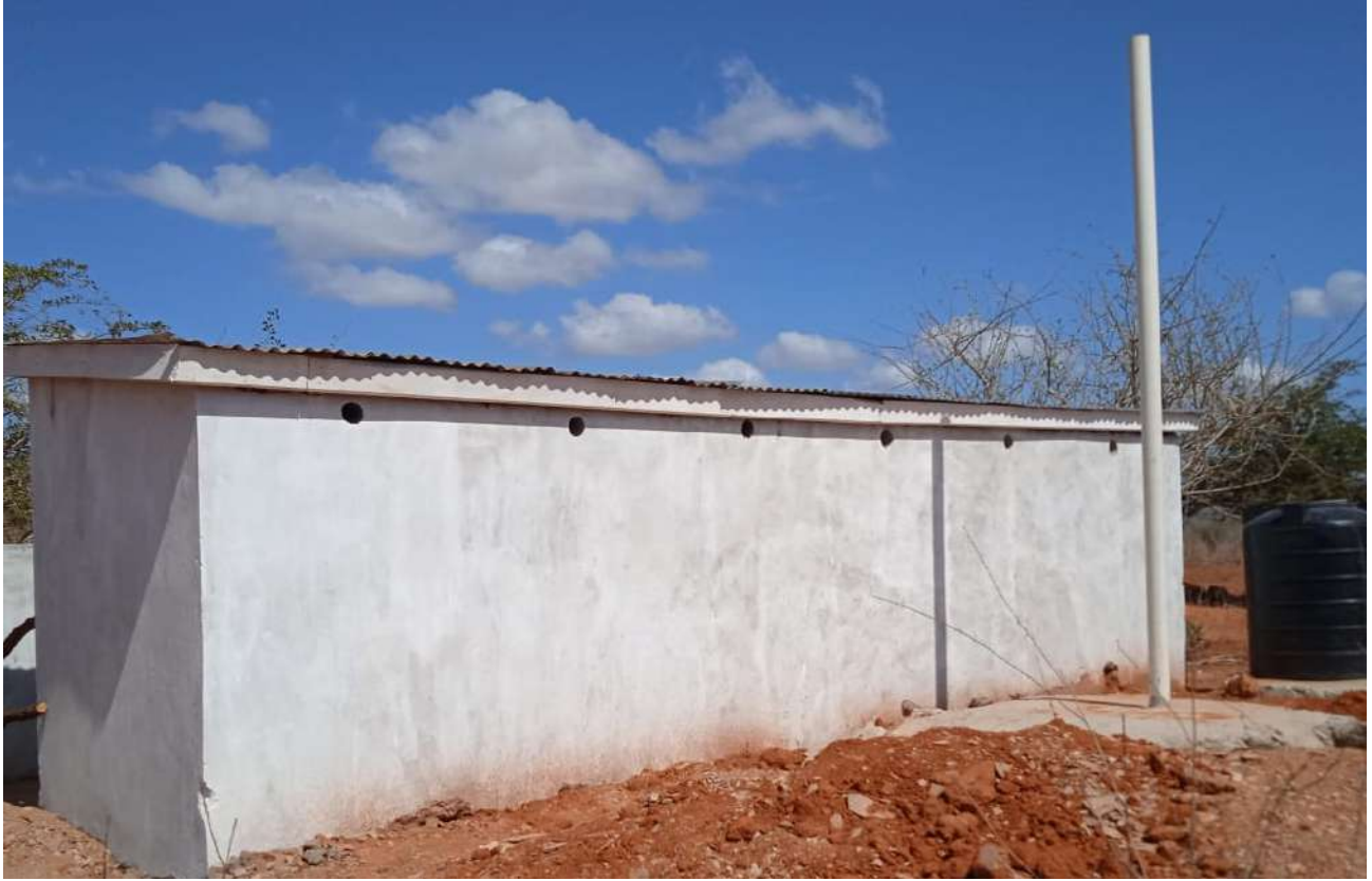
Each cubicle is individually ventilated and the pit has a long vent pipe to prevent bad smell and flies
