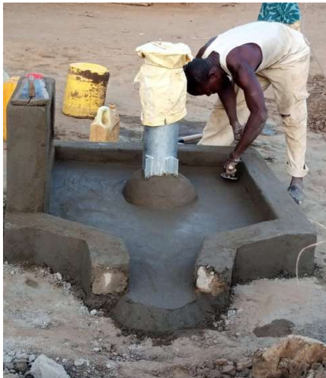
Capping, plumbing and trough completion
