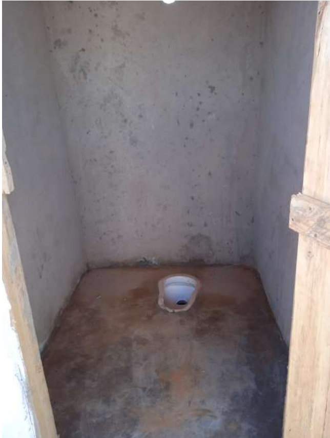
Interior of the toilets
