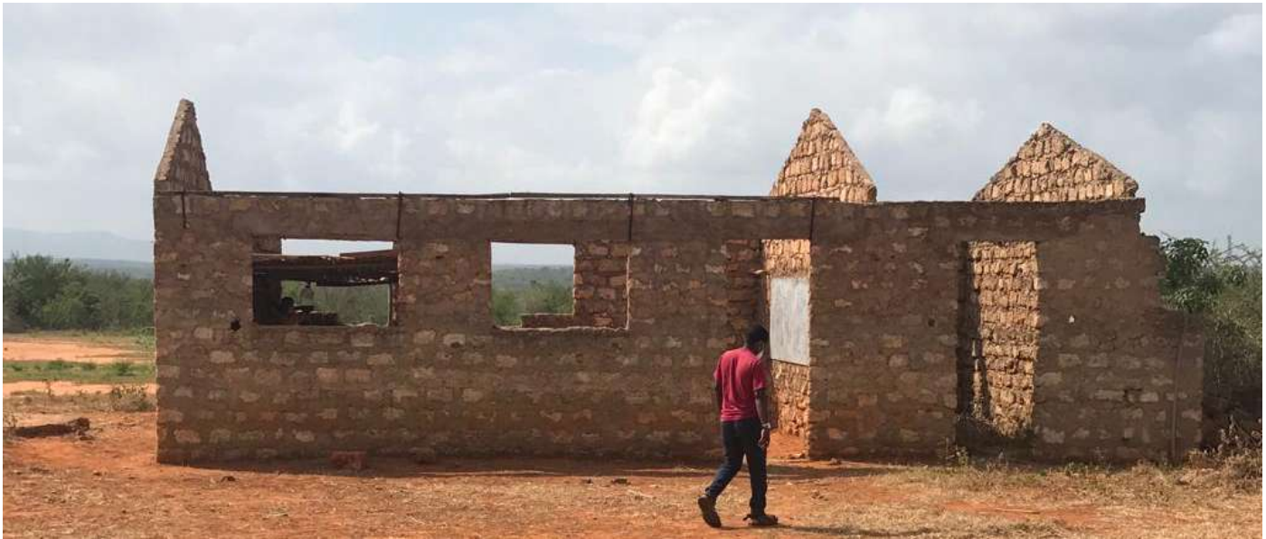
The incomplete classrooms
